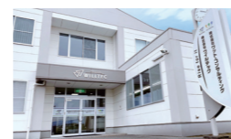
Kumamoto Technical Center (Koshi-shi, Kumamoto, Japan) Floor space : 382㎡ (two-story)
