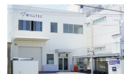
Moriguchi Factory (Moriguchi-shi, Osaka, Japan) Factory area : 907.2㎡ Equipment : General-purpose lathes, melting machines, forklifts, general-purpose milling machines, CAD, various cranes ×3, air, chiller, all types of tools
